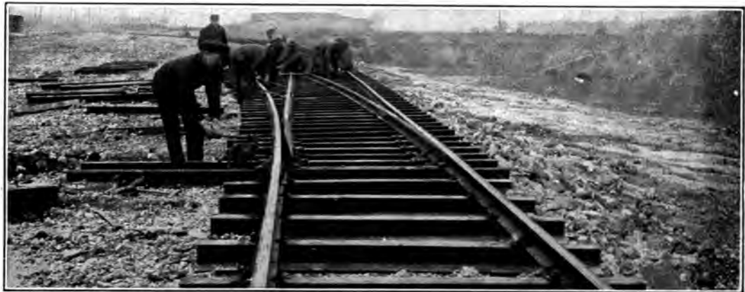
Installation Steel Switch Ties
